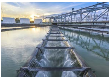
Acqua – Water treatment
